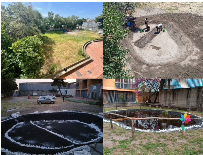
Figure 2: Pond construction timelapse
